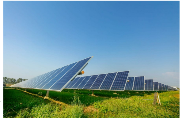
This is an example of a solar farm; source of the photo is from the Global Energy Generation website. They are the company that has proposed the solar farm that would be located on farmland east of the Bass Lake Campground.
